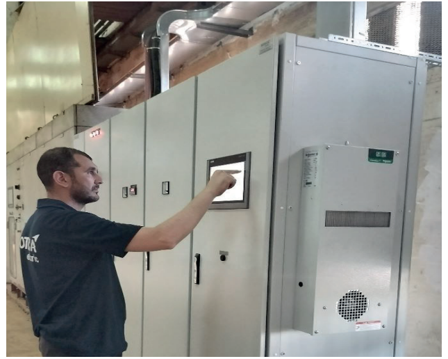
Project: Replacement of wired-logic control panels with automated-logic control panels (Tunis - Tunisia) Client: RNTA Year: 2023
