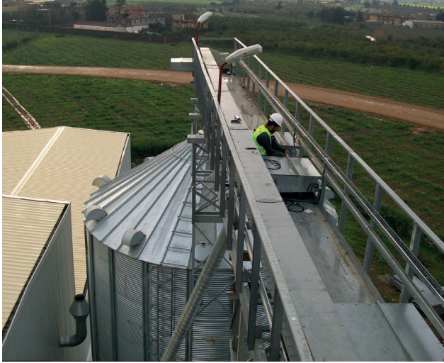
Project: Storage Center (Algeria) Client: Ounissi Brothers
