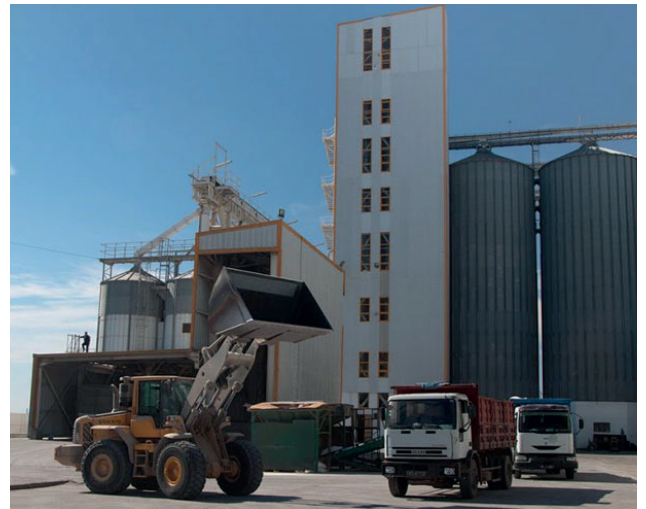
Project: Storage Center (Sousse - Tunisia) Client: Unagro
