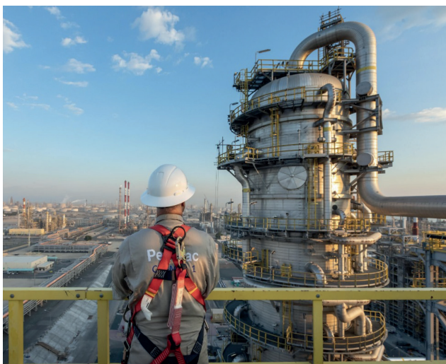
Project: Electrical Maintenance (Tunisia) Client: Petrofac
