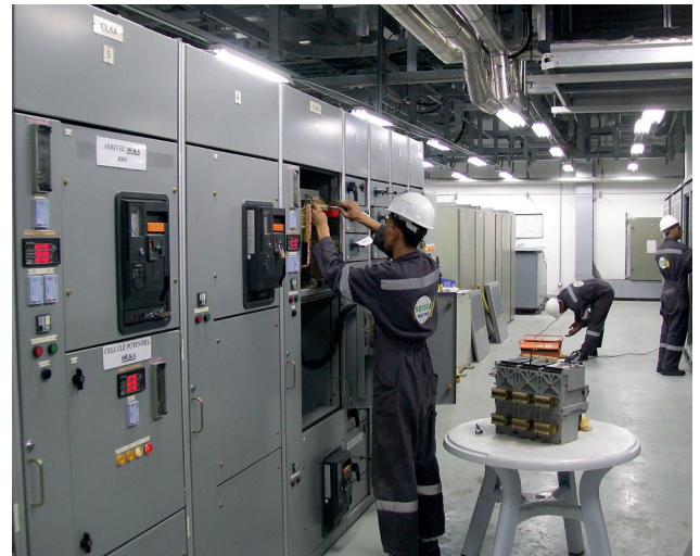
Project: Electrical Maintenance for withdrawable cabinets for a power plant (Terga - Algeria) Client: Sonelgaz
