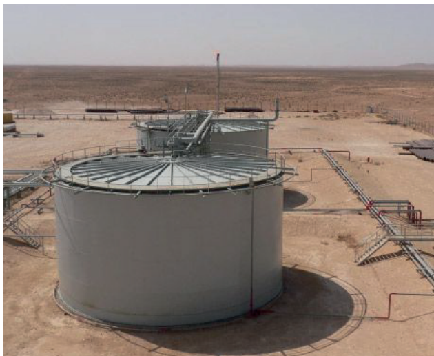
Project: Maintenance of electrical panels at the production stations in Kerkennah & Matmata (Tunisia) Client: Perenco
