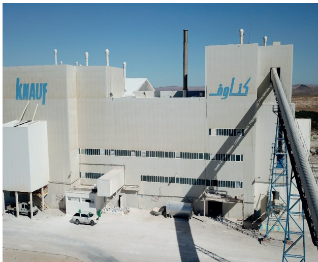
Project: Electrical Installation (Meknassy – Tunisia)
