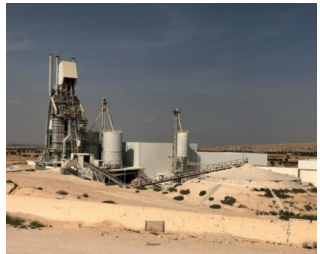
Project: Electrical installations (Gabes - Tunisia) Client: Carmeuse
