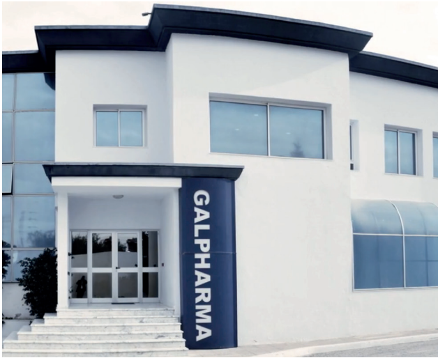
Project: Electrical installation in a Pharmaceutical Factory (Sfax - Tunisia) Client: Galpharma
