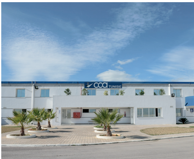
Project: Electrical Installations (Tunis - Tunisia)
