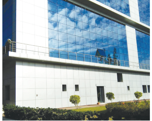
Project: Electrical installation (Algeria) Client: Industries Médico-Chirurgicales (IMC)
