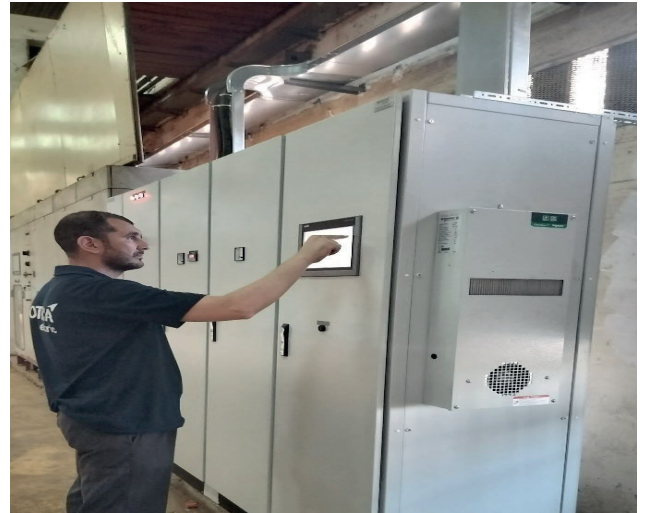
Project: Replacement of wired-logic control panels with automated-logic control panels (Tunis - Tunisia) Client: RNTA
