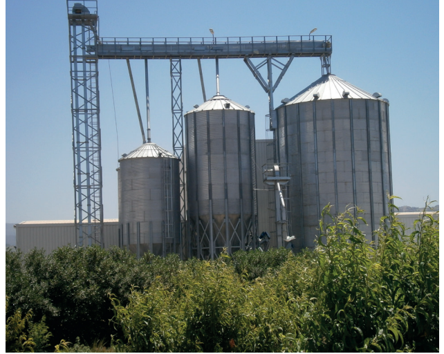
Project: Cattle Feed Factory (Algeria) Client: Khnis
