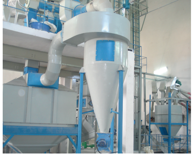
Project: Cattle Feed Factory Al-Marai (Libya) Client: Adem
