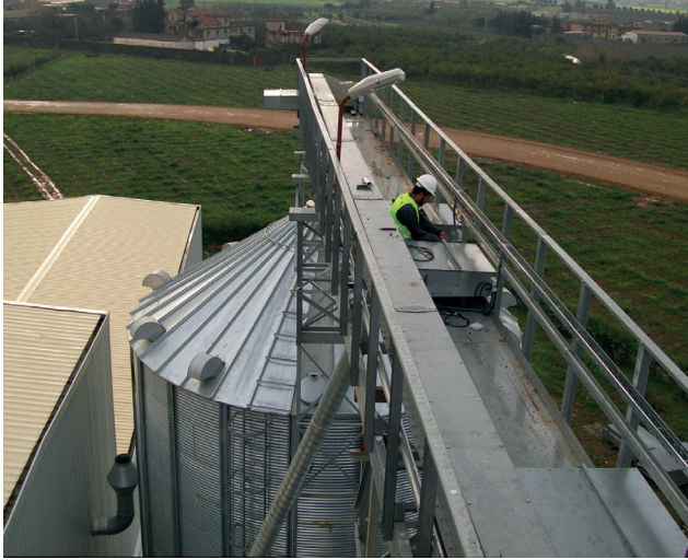
Project: Storage Center (Algeria) Client: Ounissi Brothers
