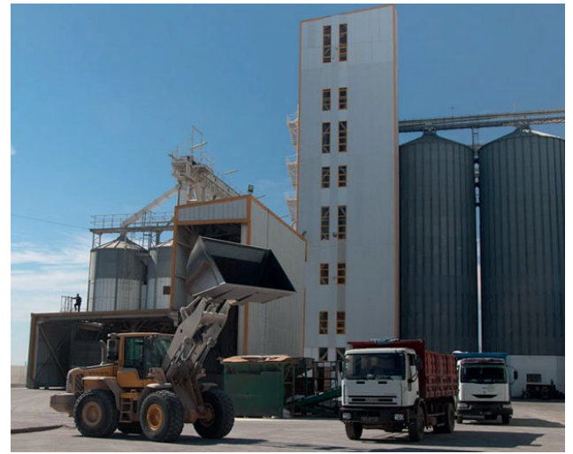
Project: Storage Center (Sousse - Tunisia) Client: Unagro
